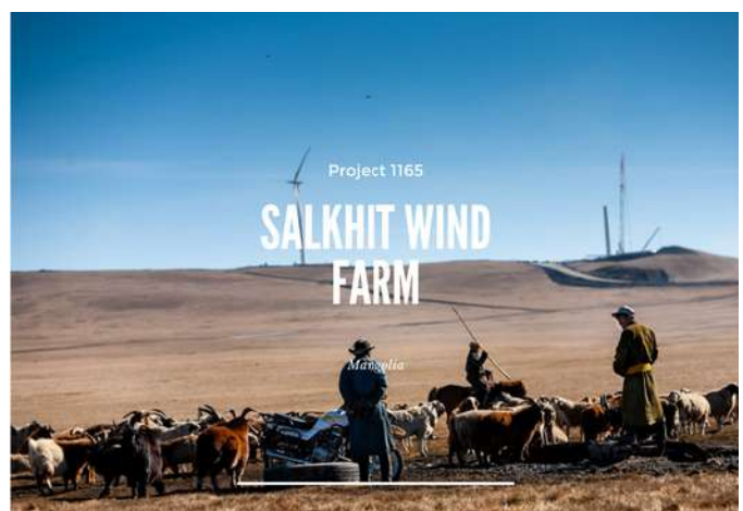
Project 1165: Salkhit Wind Farm in Mongolia
